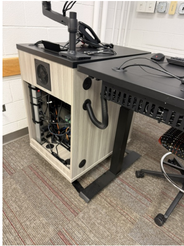
Rear cabinet access and cable routing
